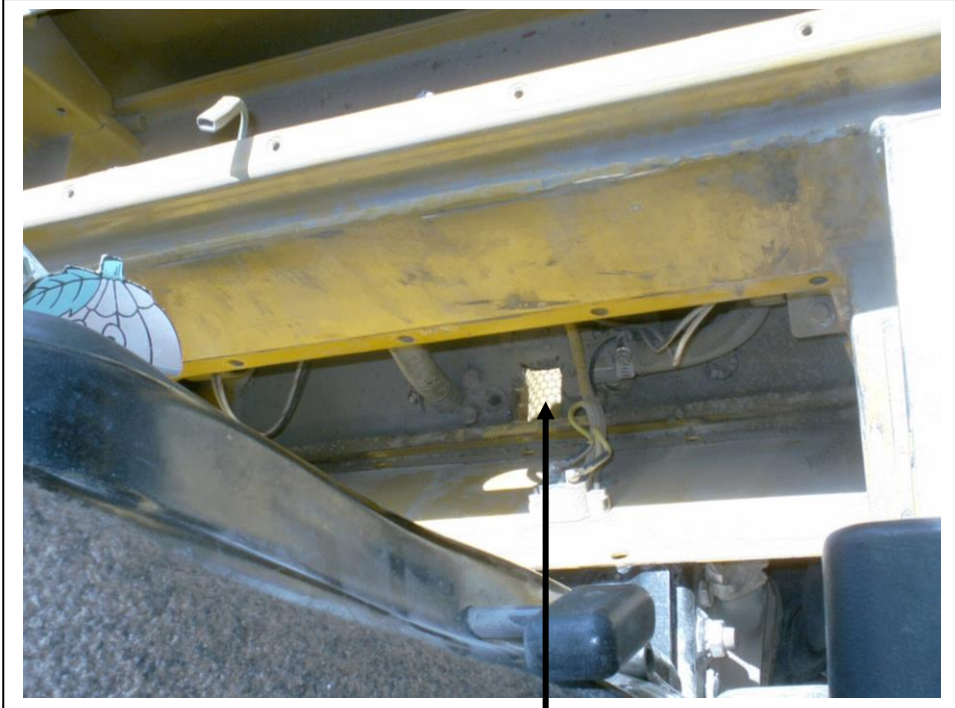
Drill, cut, chisel open this area to allow A/C hoses into the cab.
